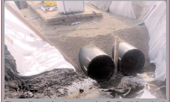
**The collapsed culvert on the Rufford Arm had to be replaced with plastic pipes**
